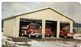
Rollins Fire Station - Built 1996
